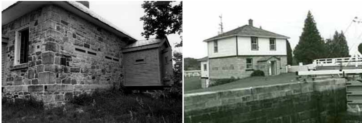
The lockmasters' houses on the Canal were made defensible with rifle slits, now often boarded or bricked up. Photos courtesy of Parks Canada.
