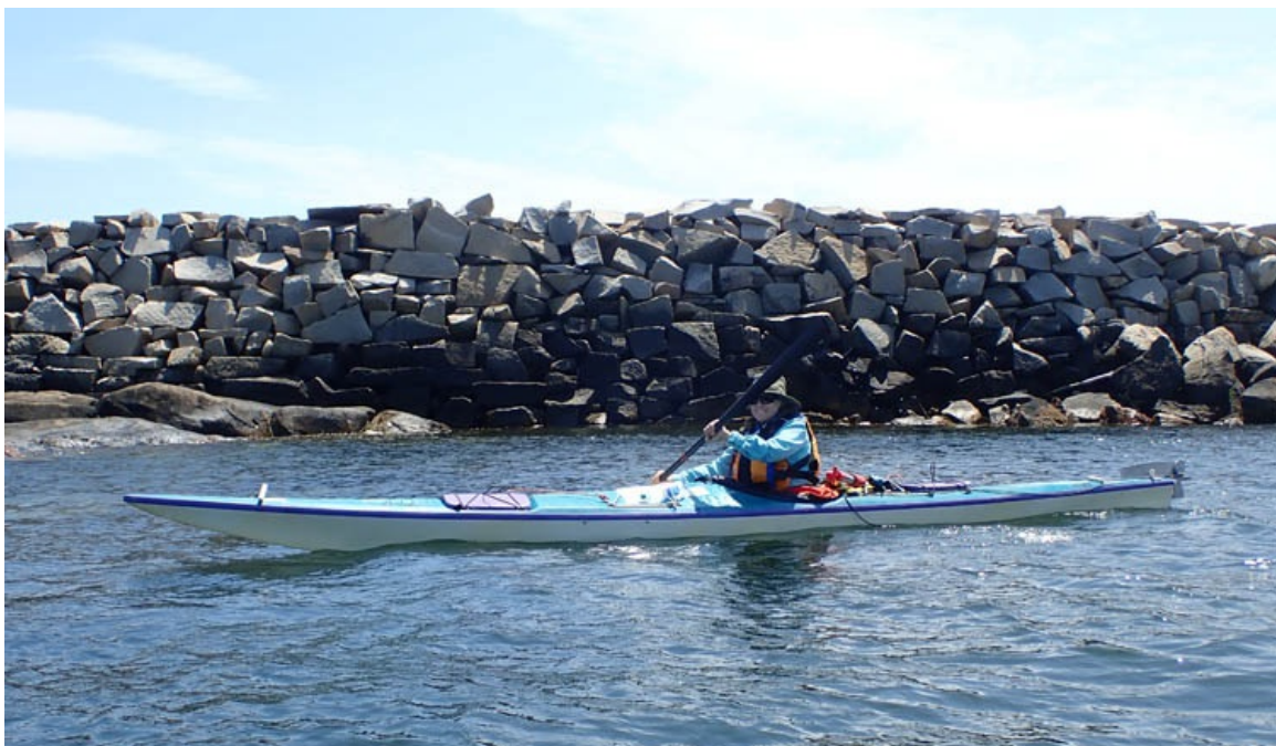
Most of the breakwater is just tumbled granite quarry waste. These piles are very common along Cape Ann's coastline.
