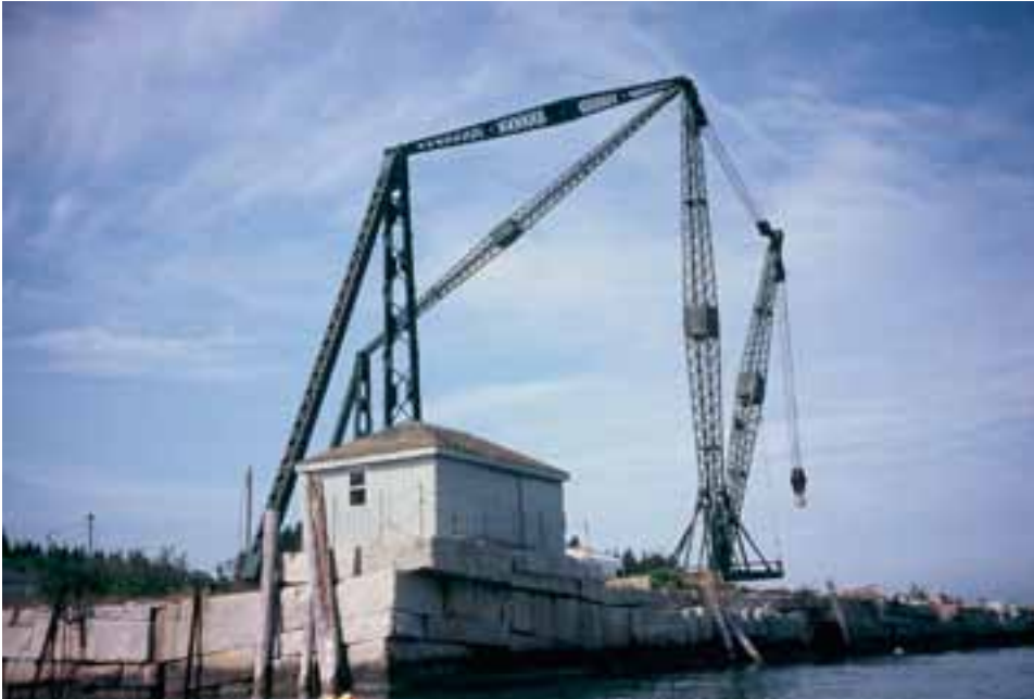
Granite loading derricks on Crotch Island off Stonington.
